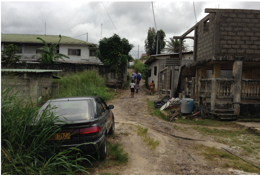
Concrete block walls and corrugated metal roof with minimal overhangs requires mechanical cooling. Ignoring the climate is neither Lean nor comfortable.
