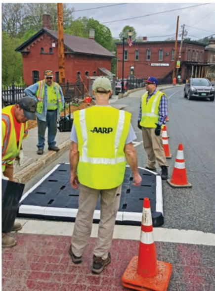
◀ MAIN STREET, BETHEL, VERMONT: During the Bethel Better Block pop-up demonstration event in 2016 (far left), bulbout curb extensions were crafted out of straw-filled wattles encircling potted plants. Soon after, rubber bulbouts (left) were installed along the roadway.
